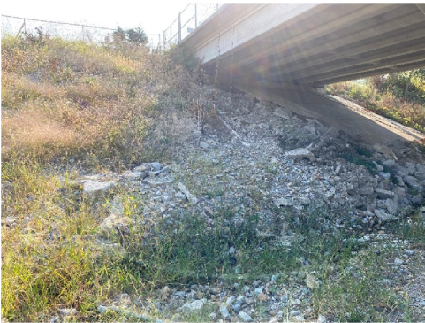
Deteriorated East Abutment Slope Protection
