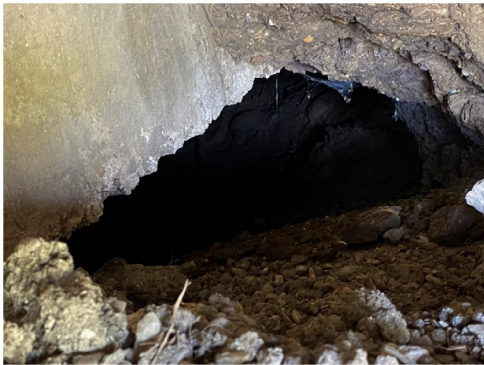
Void Under North End East Abutment
